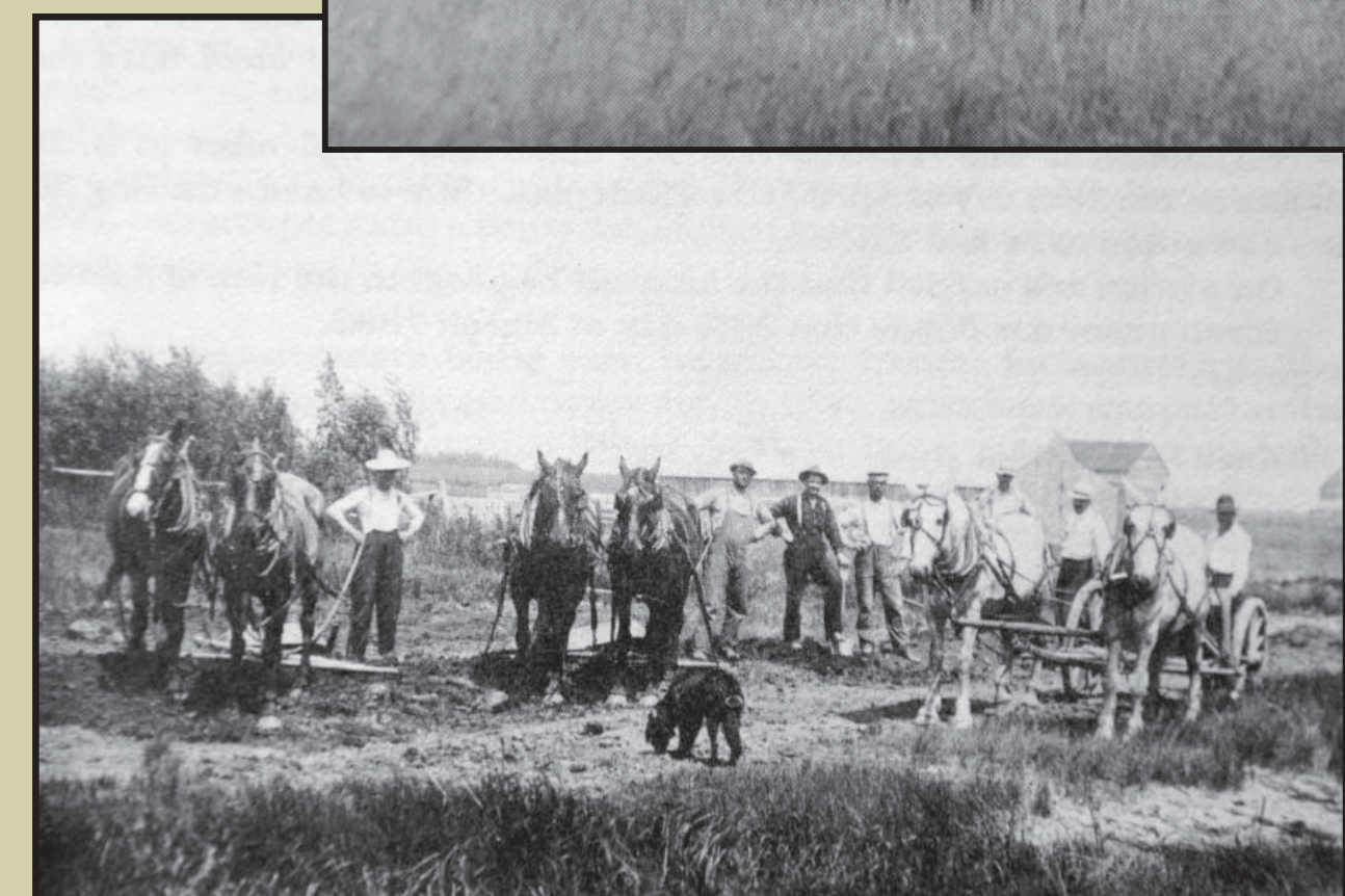
Above: A typical mode of transportation in the 1800s. Below: A road building crew in New Folden Township. Circa 1890s.
