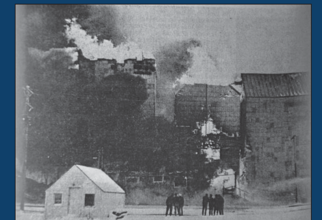
The fire in 1972 was thought to have started in the office area.
