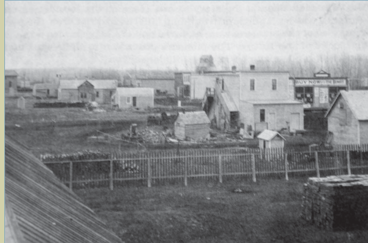
Looking east from the roof of the Bovey Shute Lumber Company. The Newfolden Post Office is the largest building at the center left.
